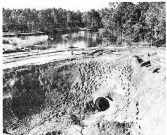
Figure 13. Test 4 of bolted 1.25% fiber module - exterior berm before the shot
