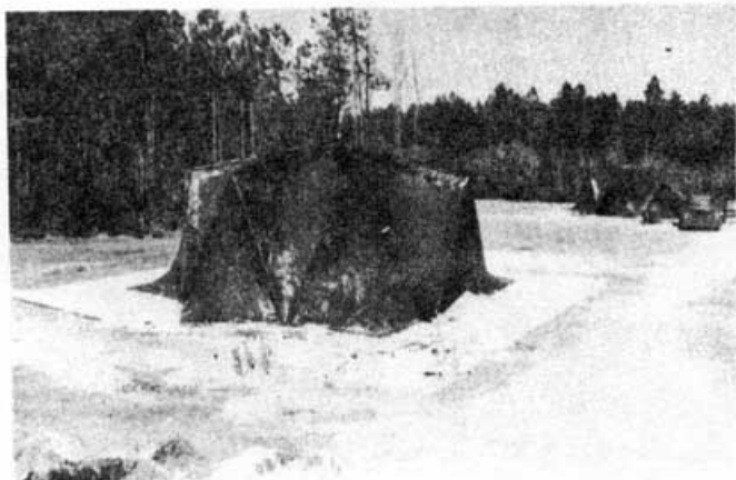
Figure 11. Both modules in place before berming
