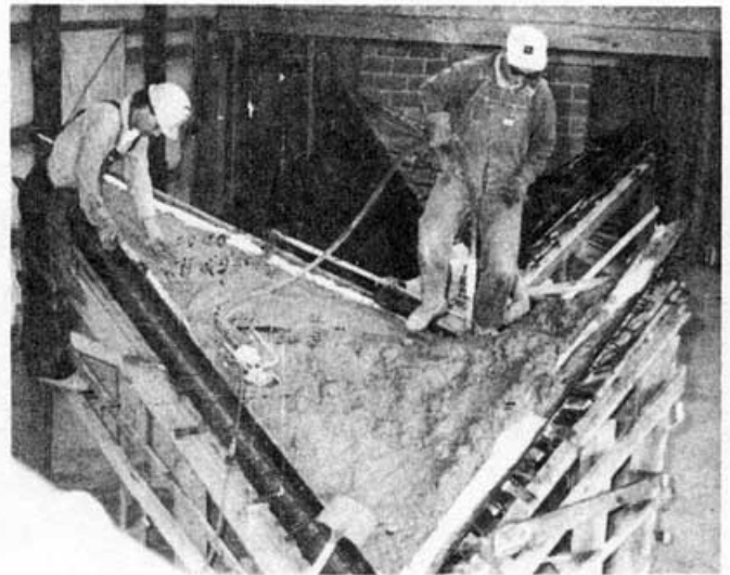
Figure 9. Placing and compacting concrete in base panel form
