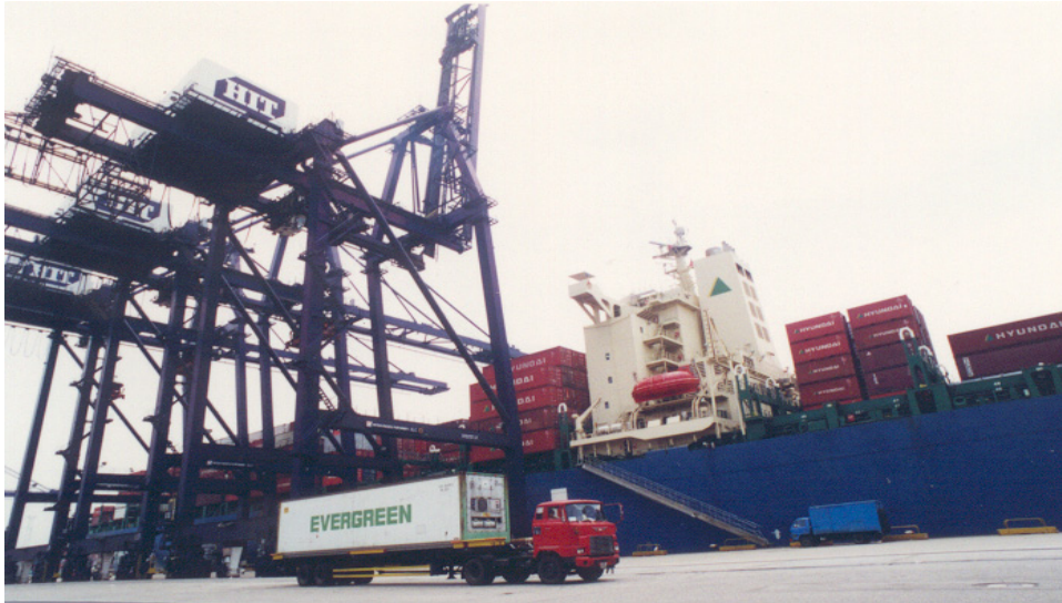
Figure 3. A QC with an IT serving it. A vessel docked on the berth can be seen. The QC unloads inbound containers from the vessel and places them on ITs, which take them to the storage yard for storage until they are picked up by consignees. ITs also bring outbound containers from the storage yard for the QC to load onto the vessel.
