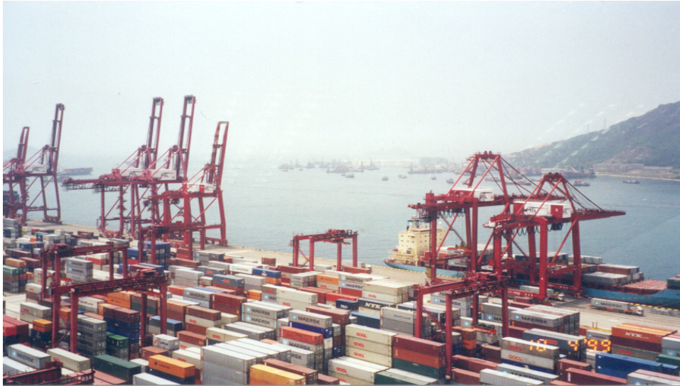
Figure 1. The container storage yard in a terminal with containers stored in columns or stacks of four to six containers. RTGCs (Rubber Tyred Gantry Cranes), which help to stack containers and retrieve them, can also be seen among the containers. The storage yard is divided into rectangular areas called blocks.
