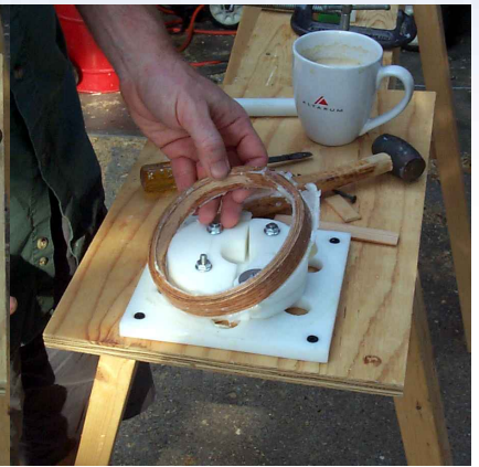
23) The hoop is free from the form and ready to be filed and sanded to finished shape. Excess epoxy will pop off the form easily.
