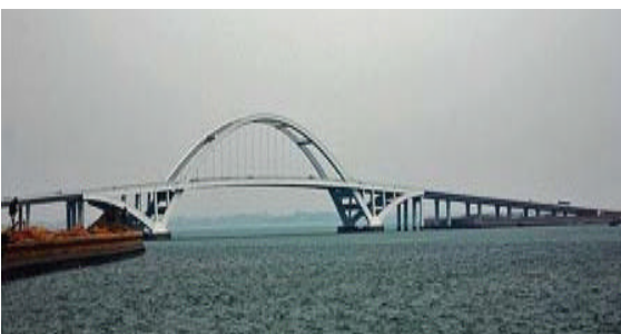
Figure 2 Side view of the Wuyuan
