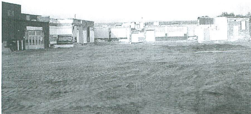
Site of New Gymnasium and Cafetorium at Onekama School
