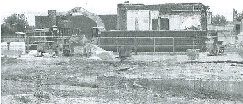
Demolition of the 1930's Onekama School for New Gymnasium and Cafetorium
