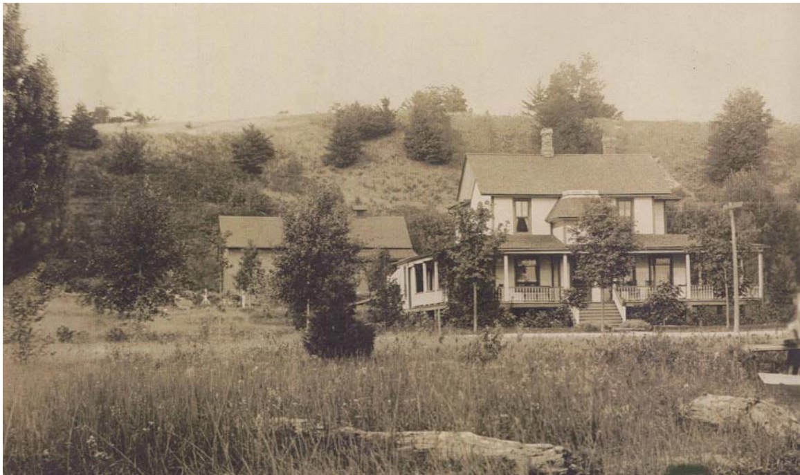
West Glenwood Building, 4594 Main Street
