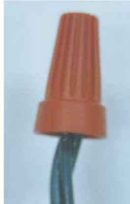
screw the wirenut onto the twisted wires
