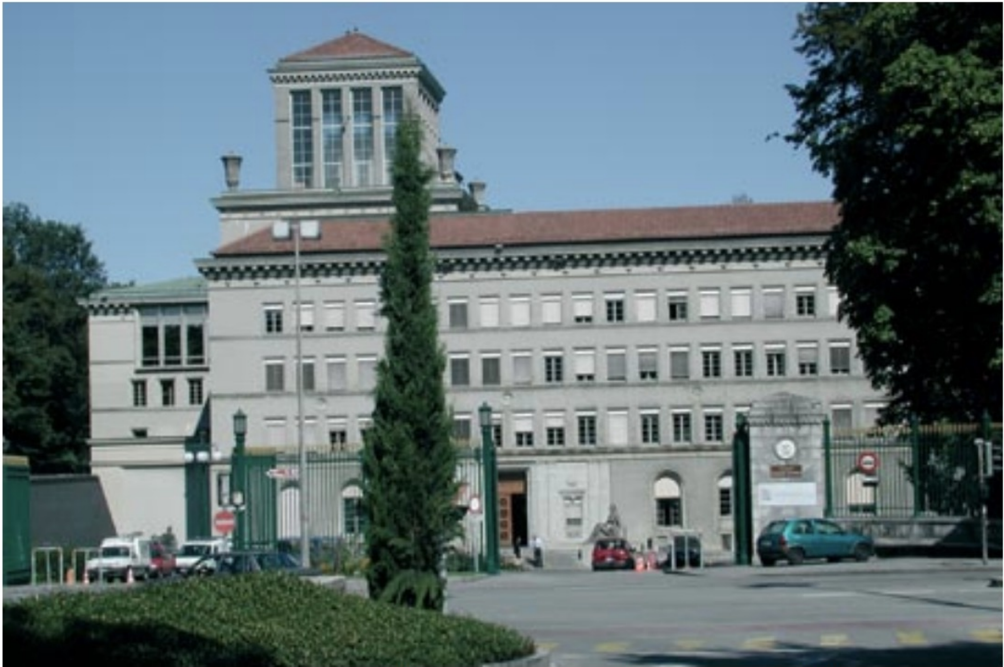
The entrance to the Centre William Rappard International
