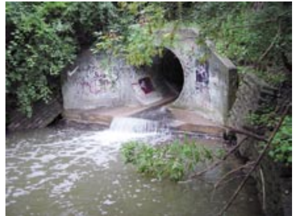
A culvert shows the size available for storm flow in Millers Creek.
