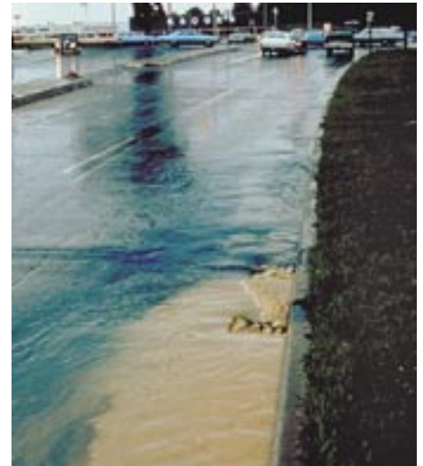
A grate in the street covers the entrance to the storm sewer.
