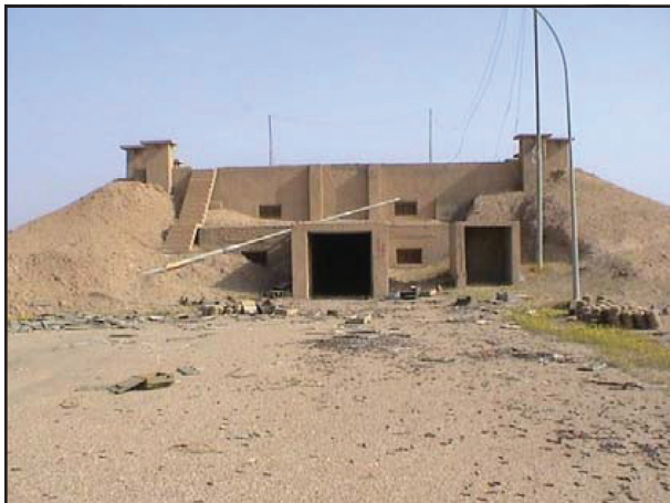
Figure 29. Small bunker with lightning protection.
