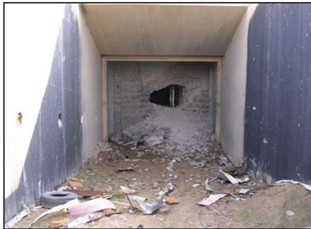
Figure 13. Bricked entryways that were breached.
